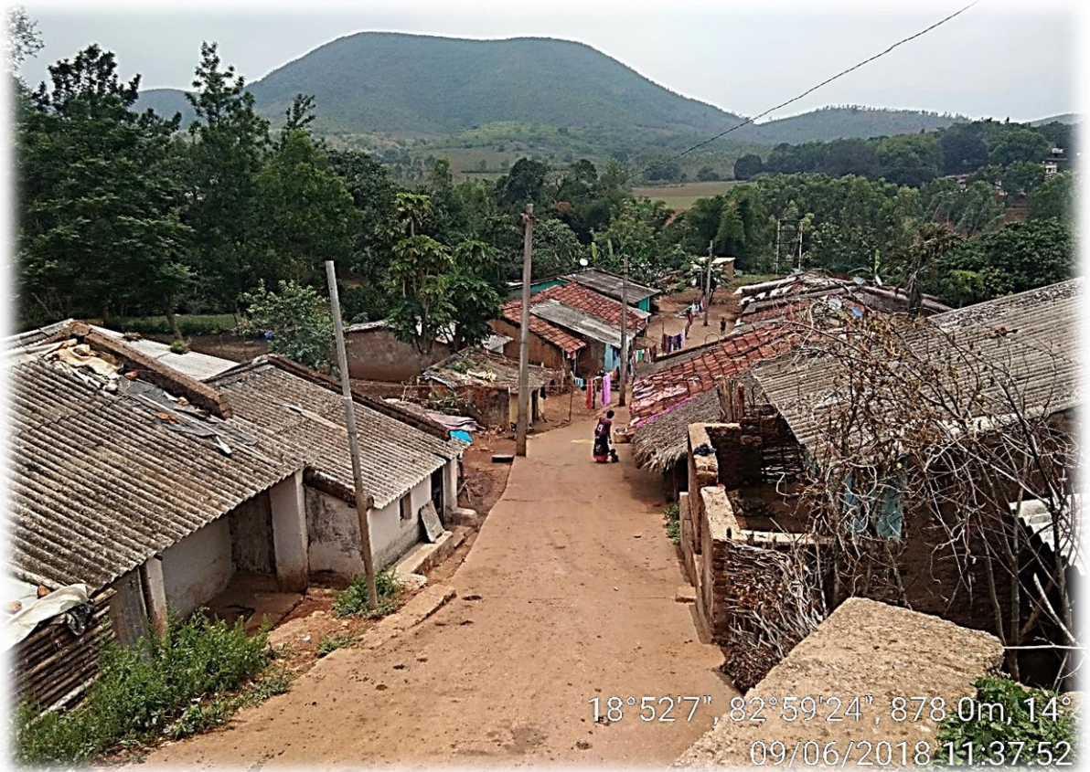
DANGAPAIGUDA ELECTRICAL PROJECT BY SOUTHCO
