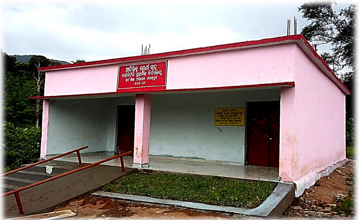
ADDITIONAL CLASSROOM AT NADIMITIKI PS NARAYANPATNA BY SSA
