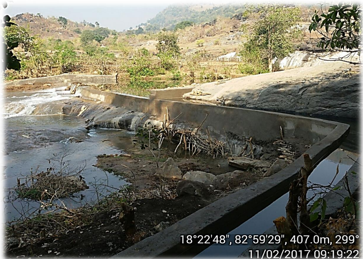
DIVERSION WEIR & FIELD CHANNEL AT POTTANGI EXECUTED BY WATERSHED
