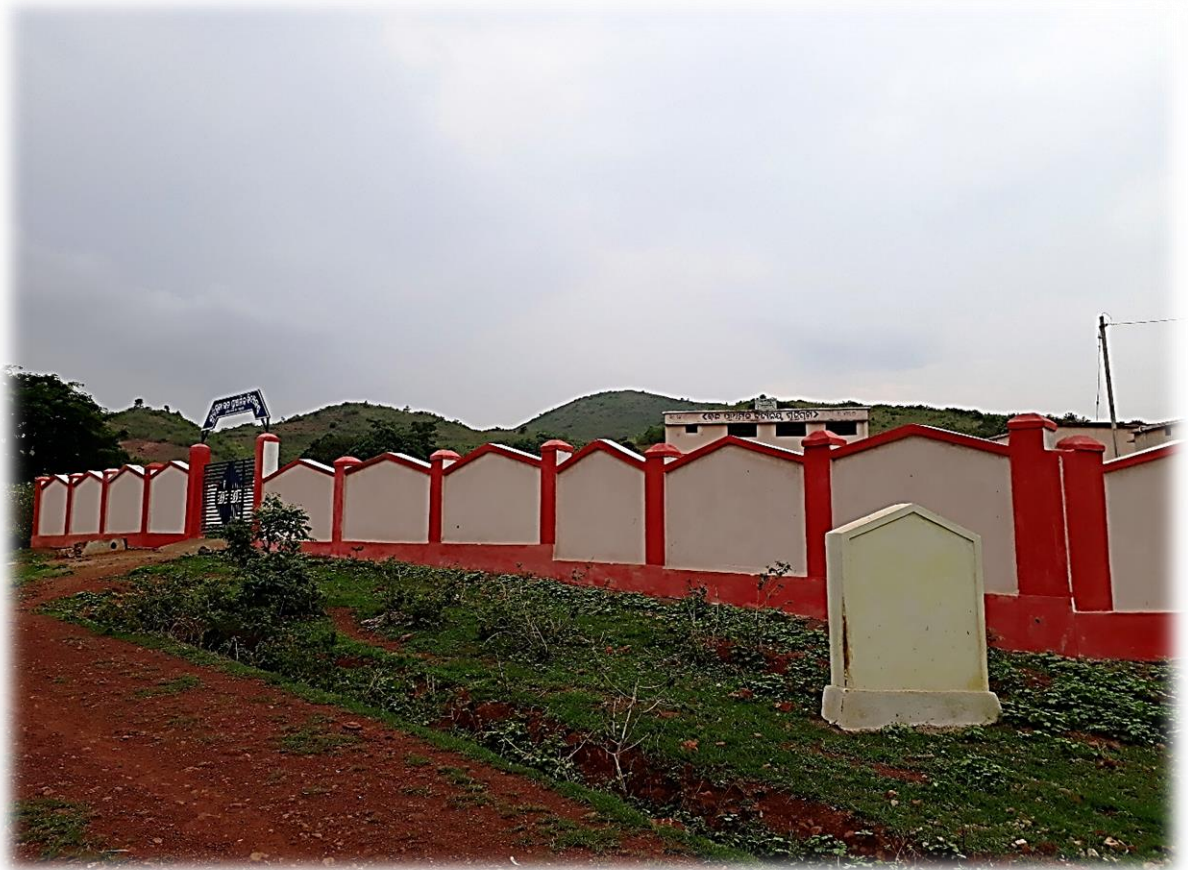
BOUNDARY WALL AT SUKRIGUDA UPPER PRIMARY SCHOOL OF DASMANTPUR BY SSA
