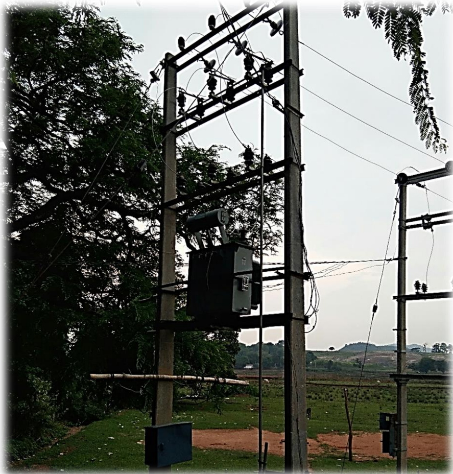
KUMARGUDA TRANSFORMER UPGRADATION WITH NEW POLE
